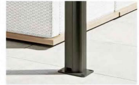
Water drop down inside the poles.
