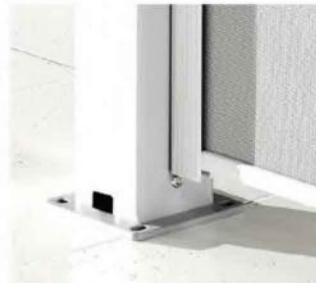
Water drainage outlet.
