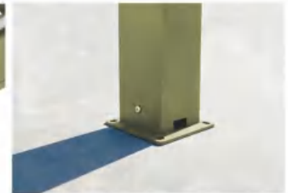
Water drop down inside the poles.
